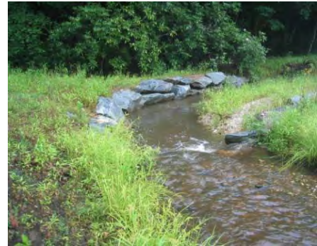
Boulder Bank Protection - Courtesy of Stantec
