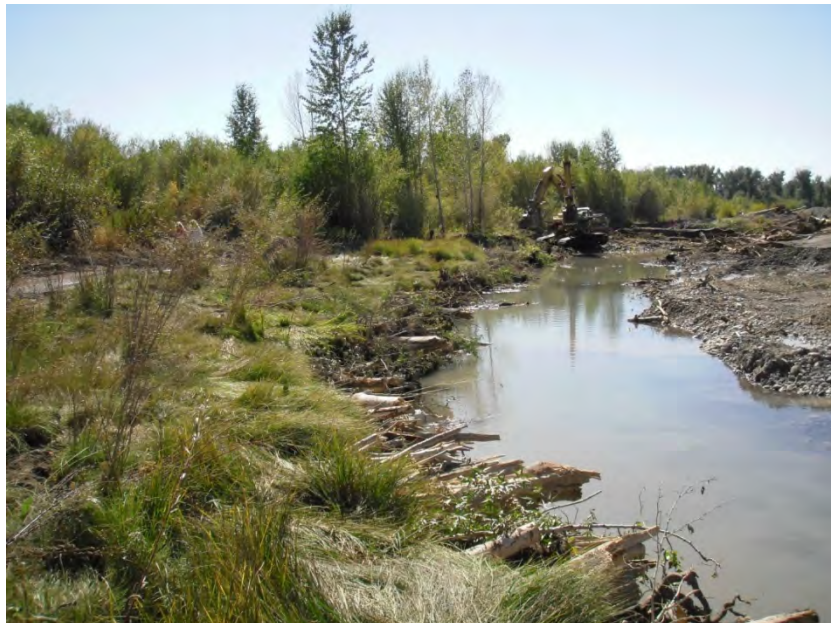
3 4 Figure 6: Woody Debris Toe Protection During Installation
