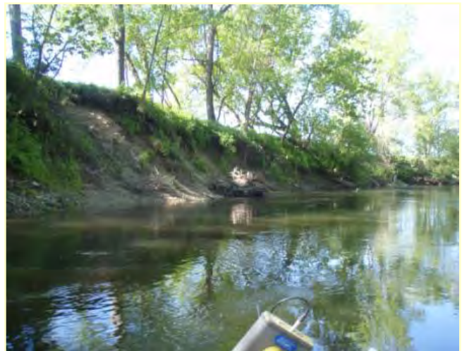
Figure 1: View of Highly Eroded Bank along the Housatonic River
