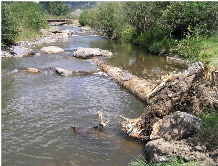
Figure 8: Example of a Log Vane
