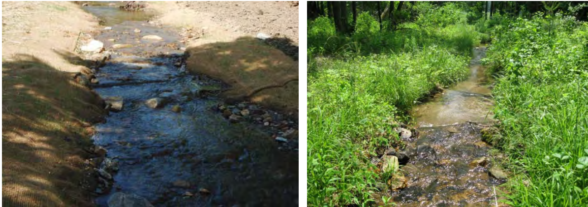
12 Figure 9: Examples of Log/Rock Constructed Riffle
